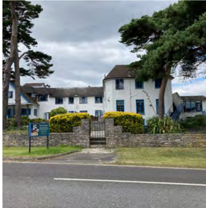
1. Existing east facade of hotel building
