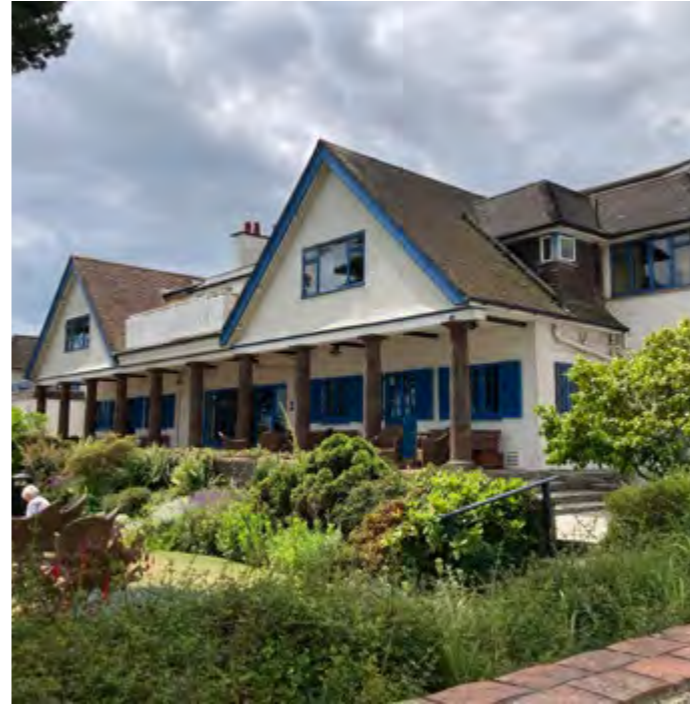
2. Mid-section of existing east facade
