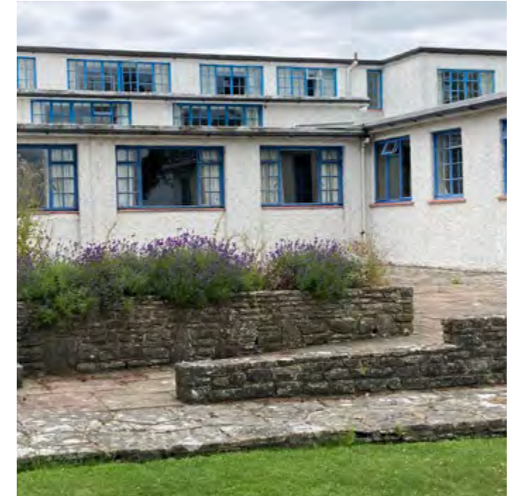
3. East facade 3 storey accommodation
